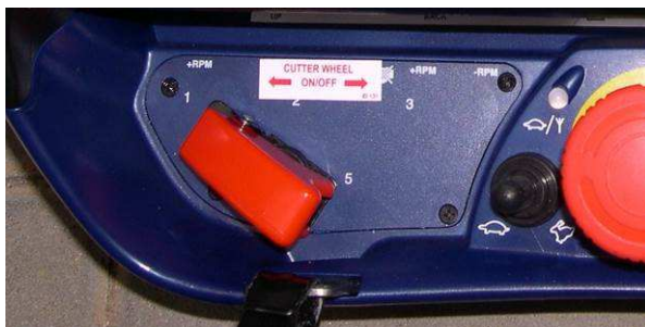
Fig. 12 – Cutting head control switch covered
